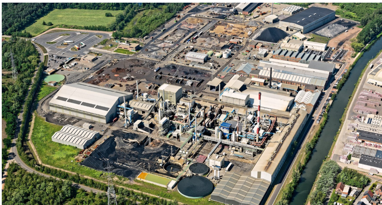
View of the Belgian site Aurubis Beerse nv, where the ASPA facility is being built
