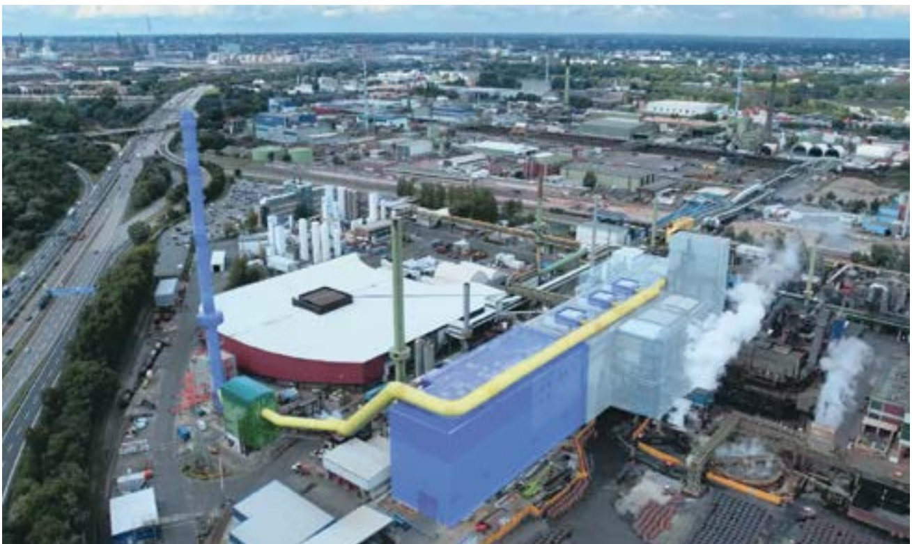
View of the new exhaust system (highlighted in color) at the Hamburg site in direct vicinity to the city
